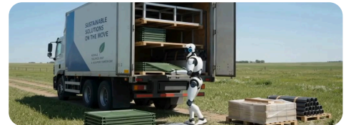
Robot-supported unloading and panel-by-panel assembly
